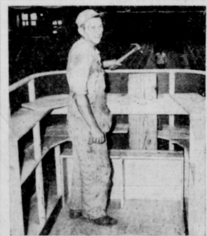
THEY'LL HEAR THAT GAVEL—Walter Fuchs is making sure that delegates to the Republican National Convention in Chicago will hear the chairman's gavel over all the fuss and furor on the floor. He's installing the 10-foot oak sounding post which will touch the floor of the convention hall and carry those rappings for order to all present.
