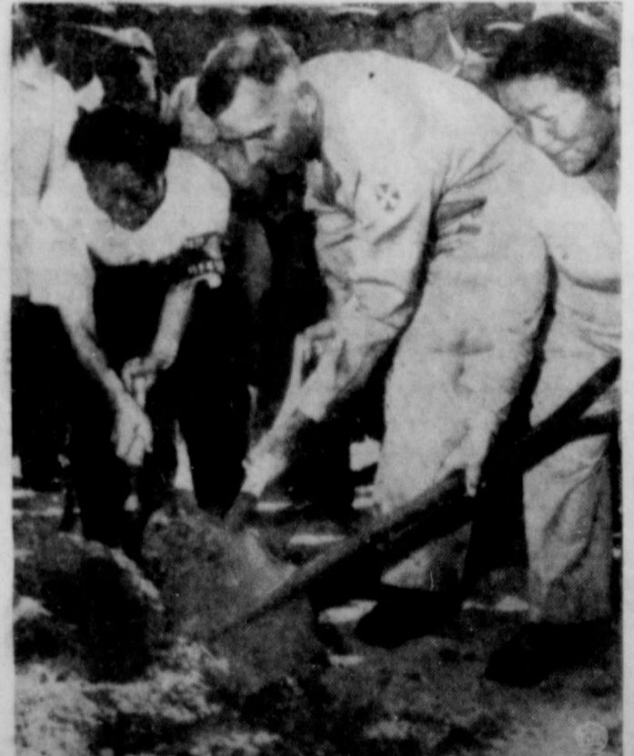
REHABILITATION PROGRAM—Eighth Army Commander Lt. Gen. James A. Van Fleet takes his turn with a shovel as the rehabilitation program of war devastated Seoul, launched by South Korean President Syngman Rhee August 21, gets under way. Gen. Van Fleet promised the Korean people the United Nations would stay in Seoul and that the old capital "will never again" be taken by the communists. (NEA Telephoto).
