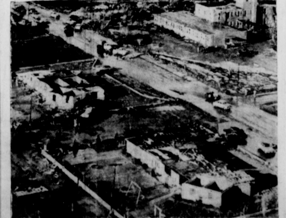
TORNADO PASSED THIS WAY —The buildings, above, unroofed, smashed and set awry are in Knox City, Tex., hard-hit by one of the tornadoes which swept north Texas and central Oklahoma. The early spring storms killed at least 17 persons, and caused millions of dollars worth of damage.
