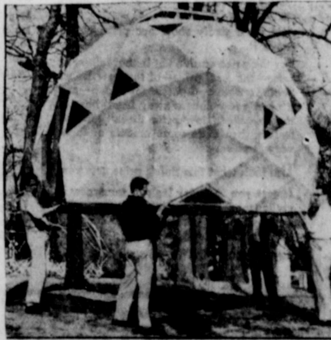
CARDBOARD VS. H-BOMB —So light that four persons can handle it, this experimental cardboard air-raid shelter is set in place on the campus at Ann Arbor by students of the University of Michigan. The collapsible, domed shelter could be mass-produced. Designer Richard Fuller believes it could better withstand h-bomb shock waves than could conventional shelters.
