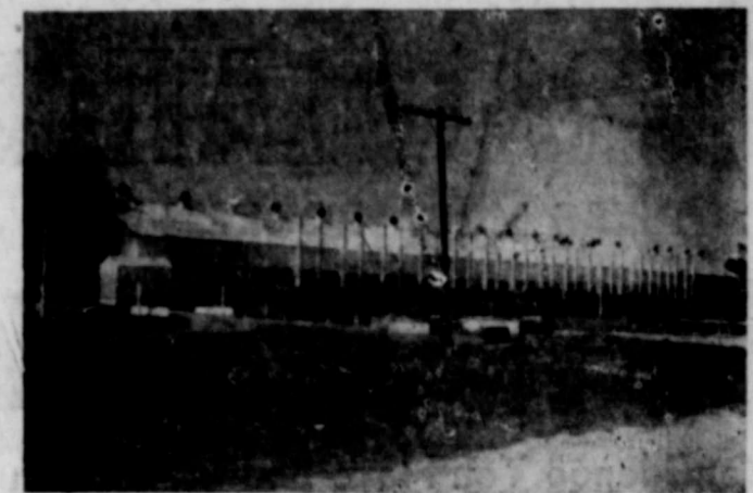
Lone Star Compressor Station No. 3
