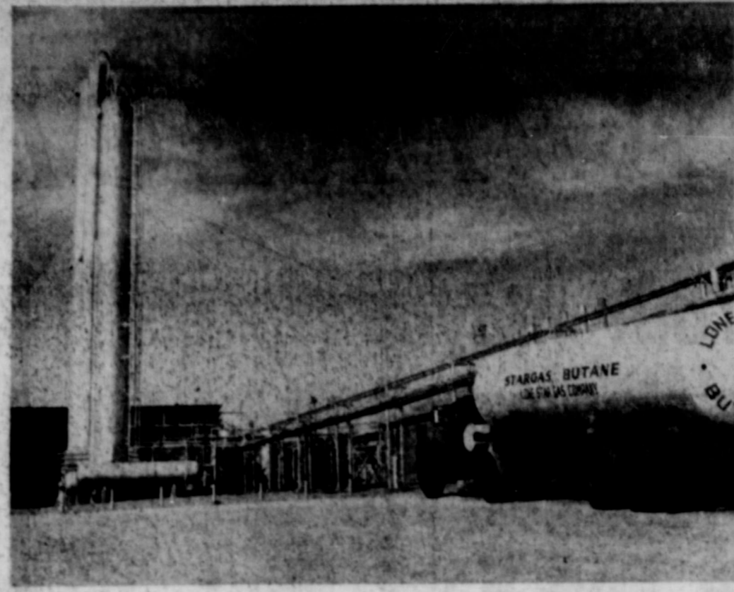
RAW CONDENSATE —A Lone Star transport truck from Gordon unloads raw condensate at Company's Ranger fractionating plant which processes hydro-carbons for shipment by tank car and truck to bulk customers. Natural gasoline is either trucked or piped to the plant from casinghead gasoline plants in the West Texas area.
