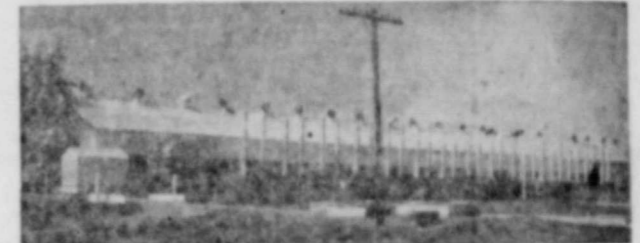
Lone Star Compressor Station No. 3
