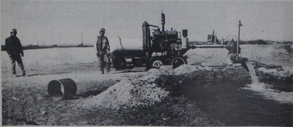
DIMMITT'S NEW WELL FIELD located about six and a half miles south of town, is getting nearer to completion with two wells in pumping condition and the other drilled. The first well drilled [in foreground] was tested at 1,000 gallons per minute with the developer pump, which will soon be replaced with a regular pump capable of bringing 650 gallons per minute to the
