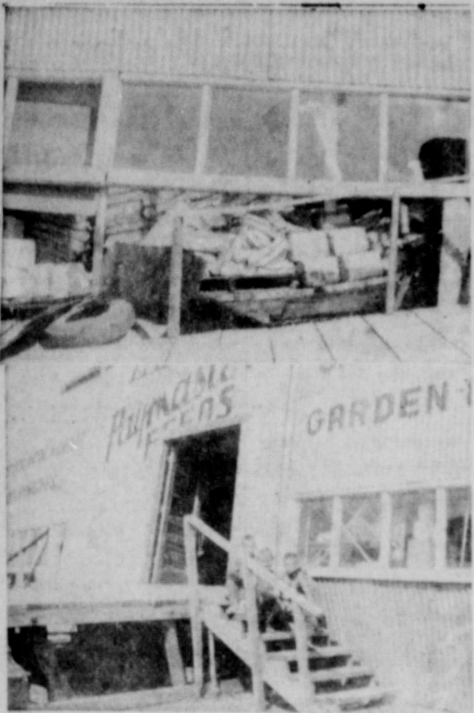
LATE SUNDAY night the floor of C. P. Cloud & Son and Rippey Bros. warehouse, 210 S. Rusk, Ranger, collapsed under the weight of about 500,000 pounds of mohair. Photos above show how the building was pushed out. Damage was extensively heavy but warehouse and contents was covered by insurance.
