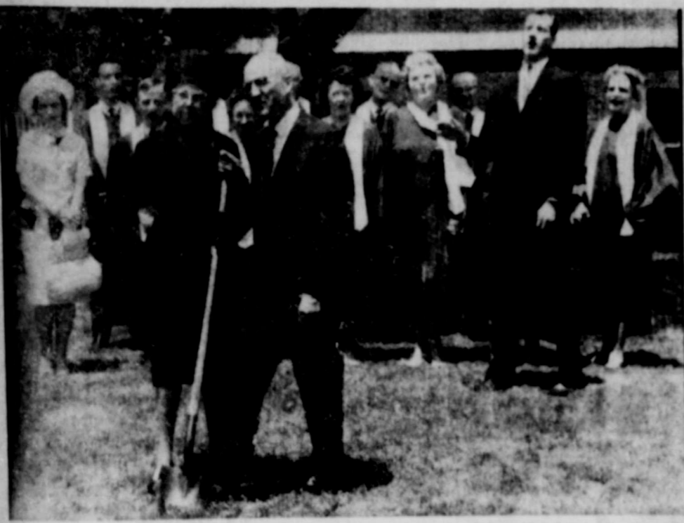
GROUND-BREAKING ceremony for Ranger's new $70,000 First Baptist Church building was held on the site Sunday morning. Oldest members of the church — in terms of service — turn the first spade of earth. They are Mrs. H. G. Adams Sr., left, and W. A. (Tony) Lewis, right. Members of church choir are shown in background. (Ed's Photo)
