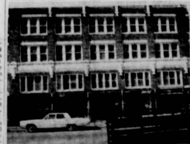
DOWNTOWN DORMITORY for male students of Ranger Junior College. Formerly the Joseph Apartments, the completely remodeled building will be ready for use in September.
