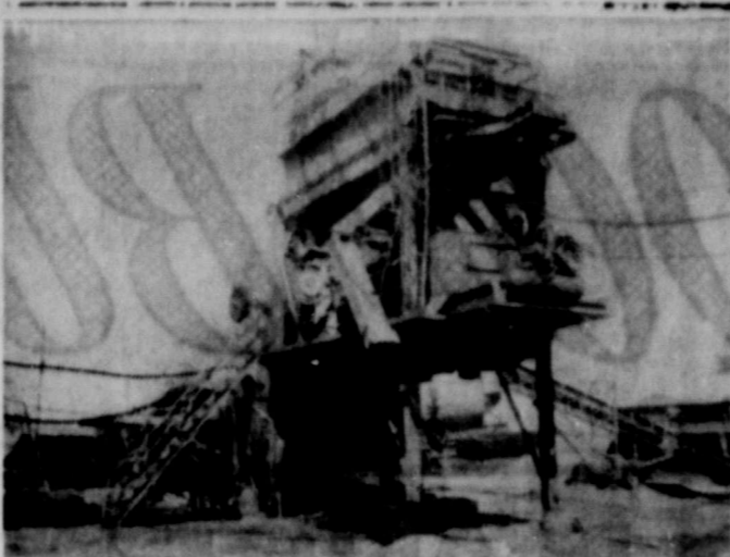
Austin Worth of Dallas has installed this Cedar Rapids hot mix Plant at the Texas Lightweight Aggregate Plant in Eastland. 6000 lbs. of hot mix can be made at one time.
