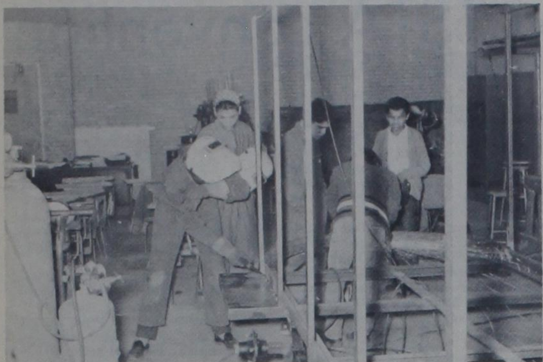
FIRST, THE FRAME — Members of Jim Dowty's general mechanics class at Dimmitt High School have just completed building — from the floor up — an all-steel custom stock trailer that includes several new innovations. Here, Robert Woolbright, George Ulloa, Joe Flores, Mike Constancio and Lino Perez weld the frame together.
