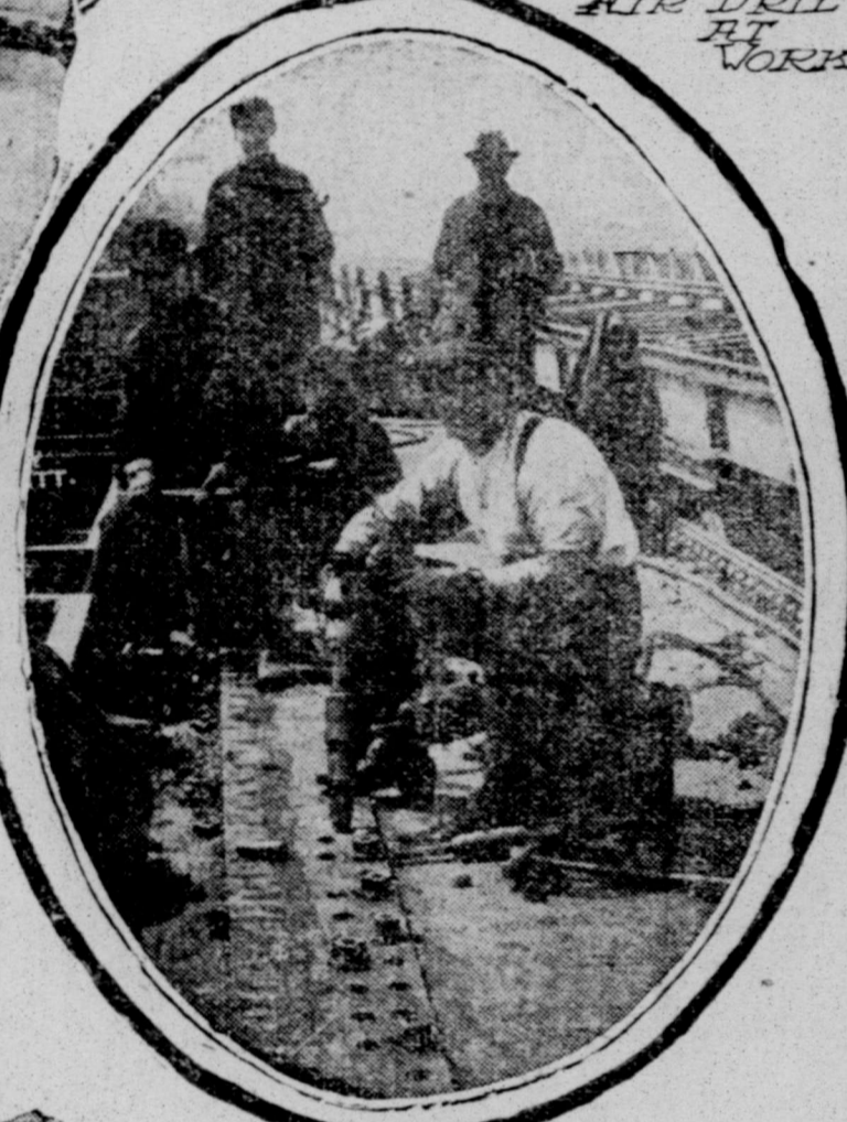
USING PNEUMATIC HAMMER IN SHIP BUILDING
