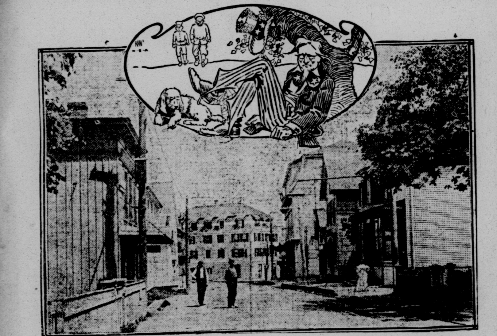
ONE OF THE QUIANT "DOWN TOWN" STREETS IN PORTSMOUTH.
