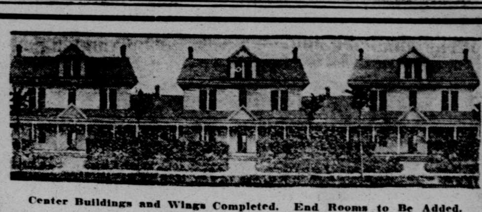
Center Buildings and Wings Completed. End Rooms to Be Added.
