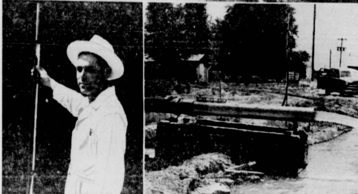
Top, testing assembly for efficiency survey on electric well at W. B. McAdams farm near Muleshoe. Shown are Jeff Peeler, Southwestern Public Service Company Muleshoe manager; Earl Lewis, agricultural engineer for Southwestern Public Service, who conceived and perfected the tester; and Warren Dayton, Lewis' assistant. Bottom left, Lewis measuring water flow through water gauge tube, and, at right, side view of water flowing through tester.
