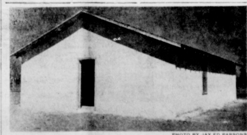
Pictured here is the 24x40 foot building recently completed on the City Park grounds for the Boy Scouts. The building construction was sponsored by the Lockney Rotary Club.
