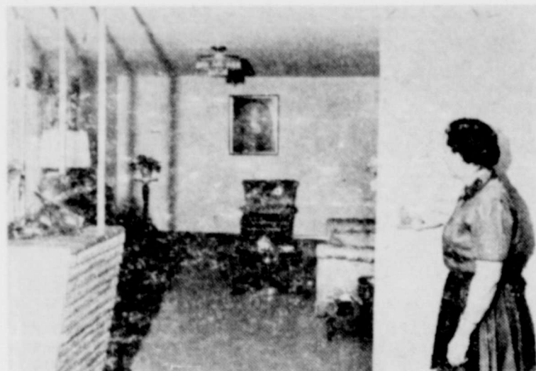
Adequate wiring lowers the cost of electric service. The Mills insisted on proper wiring. Here, Mrs. Mills demonstrates the latest in lighting switches. They're silent, working at the touch of your finger, and you always know which lights are on.
