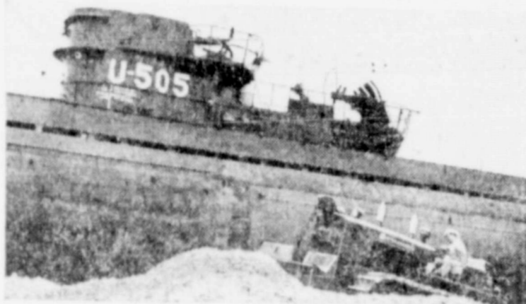
When breakers threatened to wash away cribbing supporting beached sub, International TD-24 crawler tractor was brought in, bladed sand into nine-foot-high protective dike.
