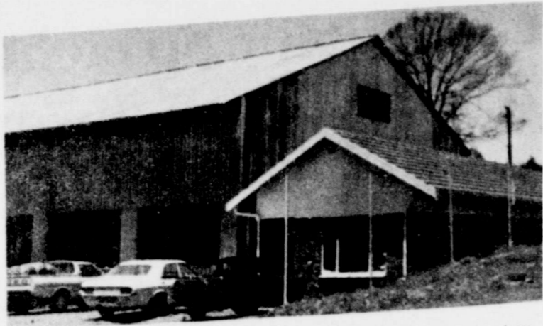
A VIEW at the new Texas Tillage Mfg. plant in the Republic of South Africa which was opened by Johnny, Willie Mae, and Mitchell Lloyd.
