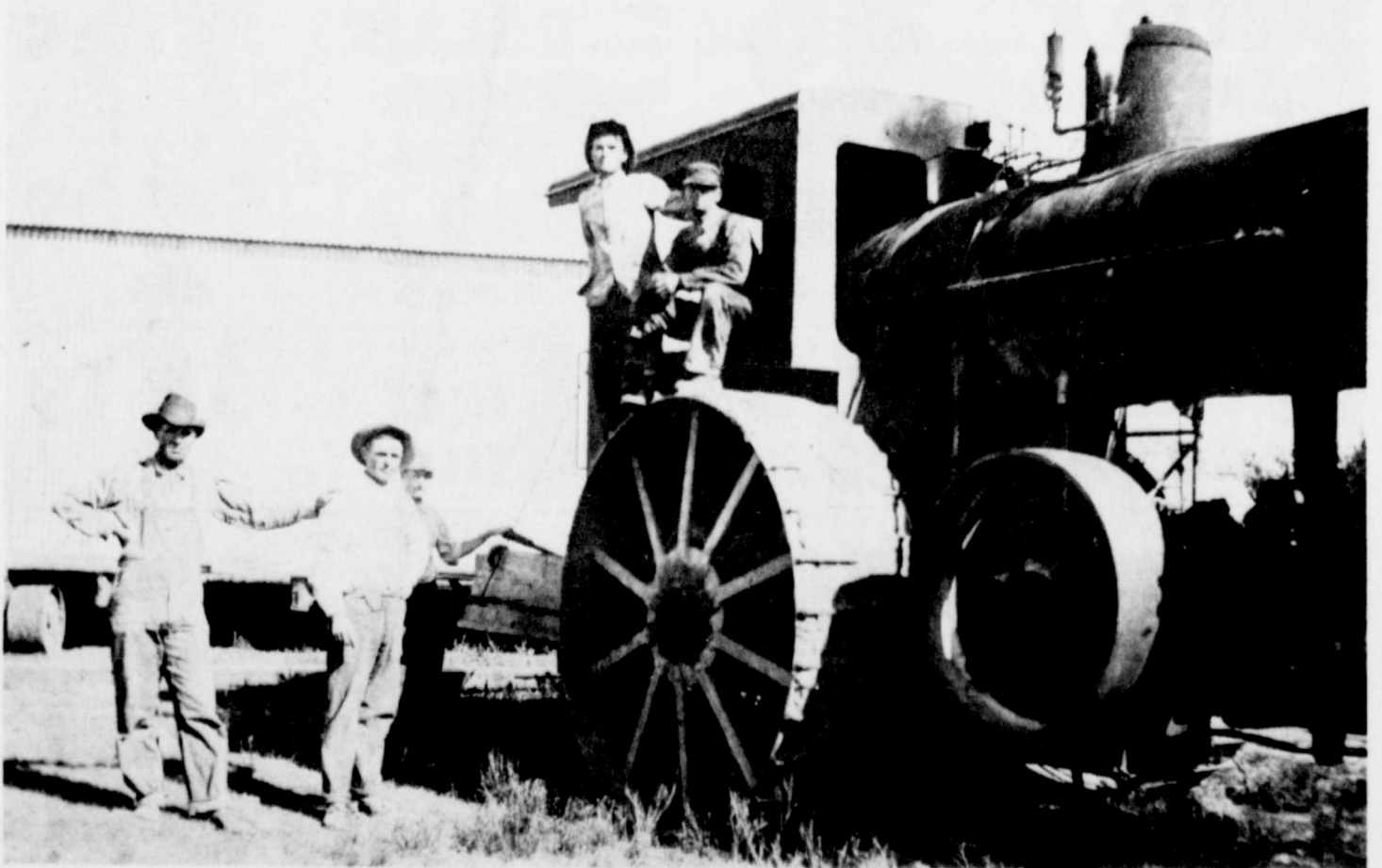
THIS OLD steam engine and trailer were used in some of Walter Byars' house moving.
