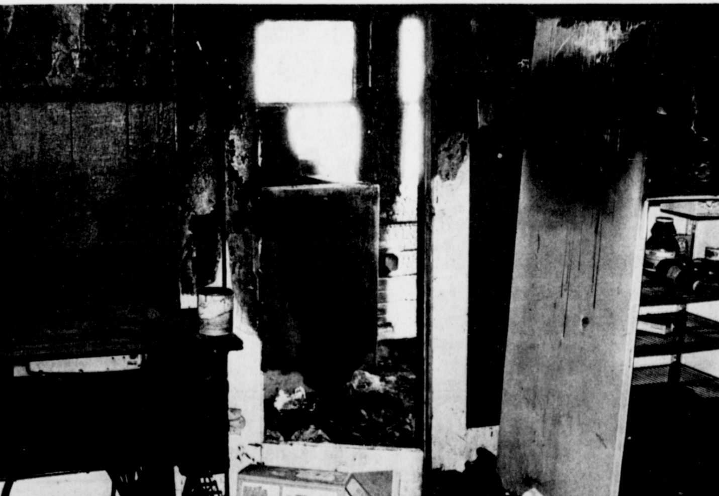
INSIDE THE STAPP HOME after the fire. (Staff Photo)
