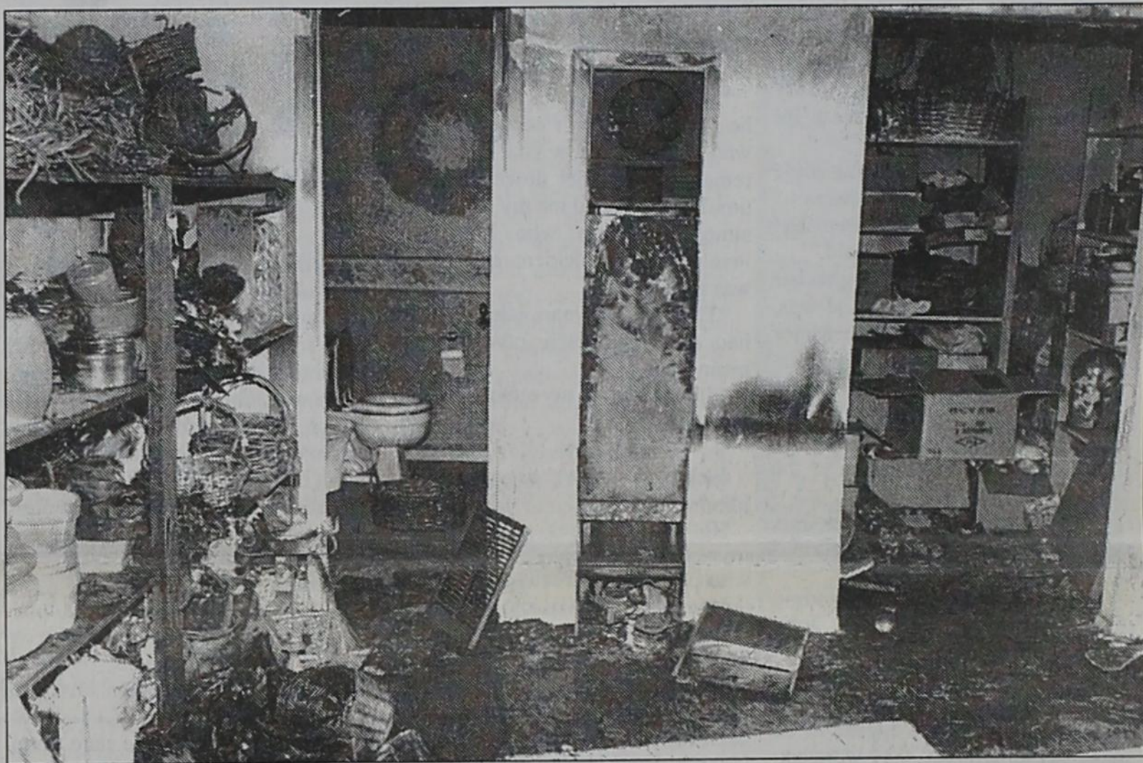
WHERE IT ALL STARTED —This wall heater in the back room of Seale Florist at 310 N. Broadway in Dimmitt is suspected to have started the blaze that damaged the business last Thursday morning. Tommy Cleavinger of the Dimmitt Volunteer Fire Dept. said something either fell or got too close to the heater. The back room was a work and storage area,
