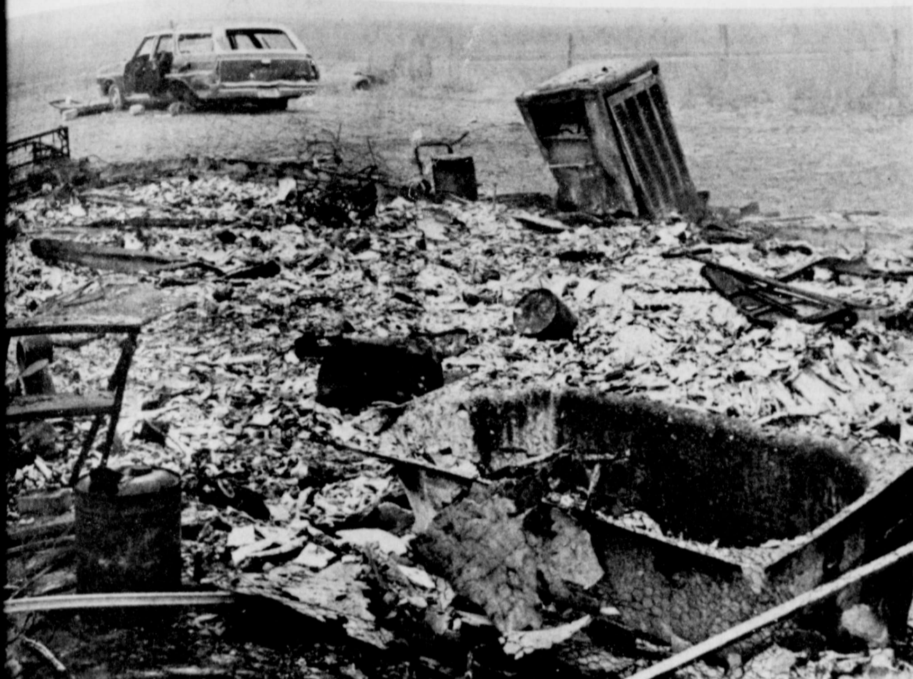
RAZED BY FIRE... A four-bedroom house stood at this site until Thursday night, when a fire destroyed the house and its contents. Also Thursday night,
