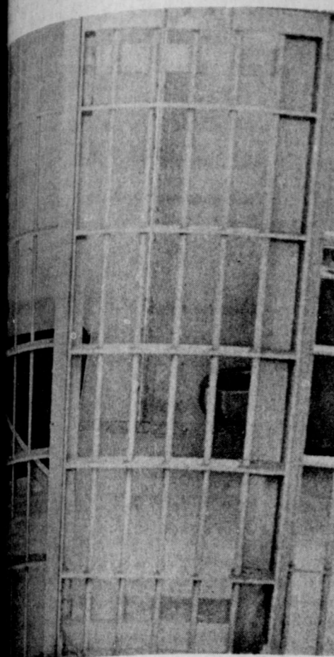
CELLS in the County Jail have a steel cot that fits the wall. The sink faucets are a push button type and the water flow. The water is heated to only 100 degrees Fahrenheit.
