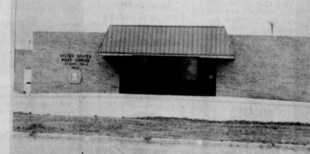
POST OFFICE nears completion.
