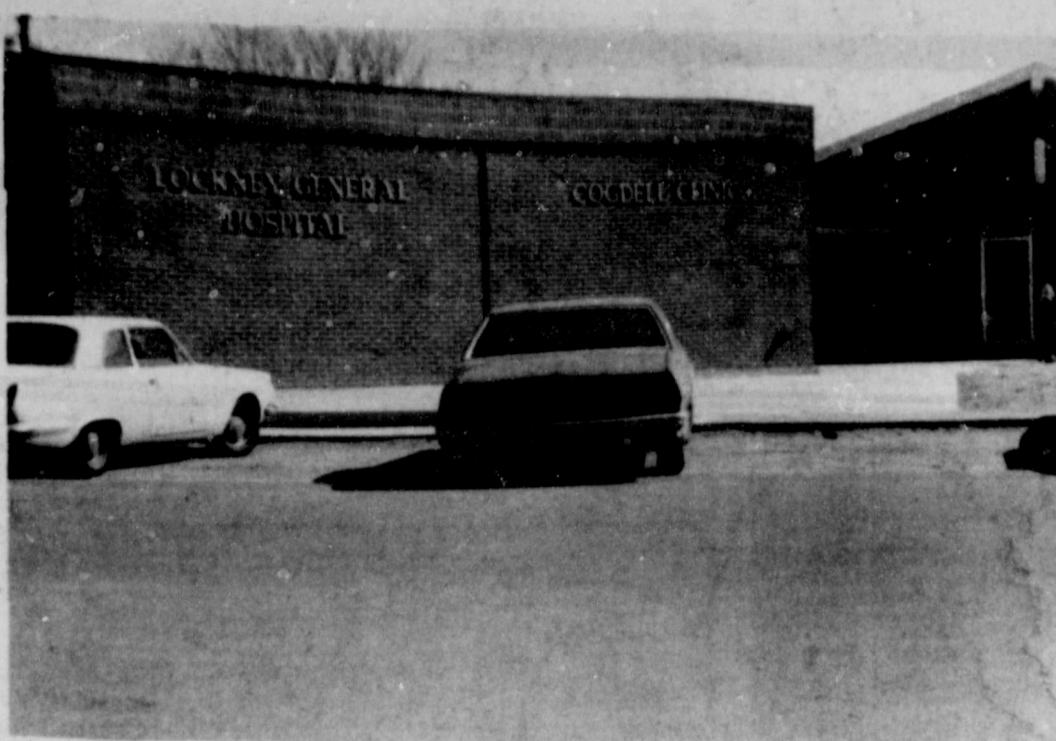
FINISHING TOUCHES were put on the Cogdell Clinic of Lockney General Hospital this week when the letters announcing the name of the clinic were put in place. The actual clinic building, the gift of the Martha Ann Cogdell family was completed in September 1980.
