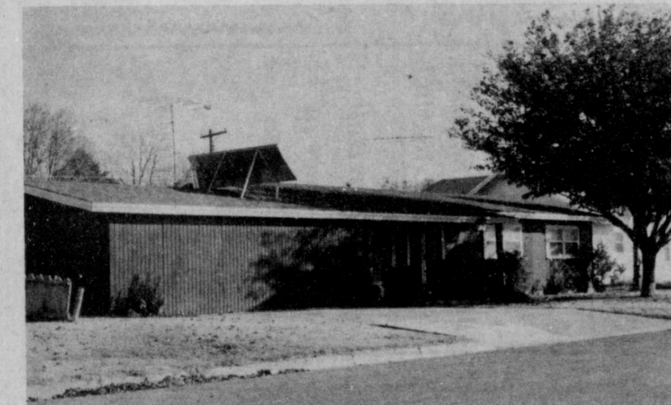
A SOLAR UNIT has recently been installed on the Billy Joe Turner residence for supplementary heat. An Open House is being held Saturday from 10-4 for the benefit of the public.
