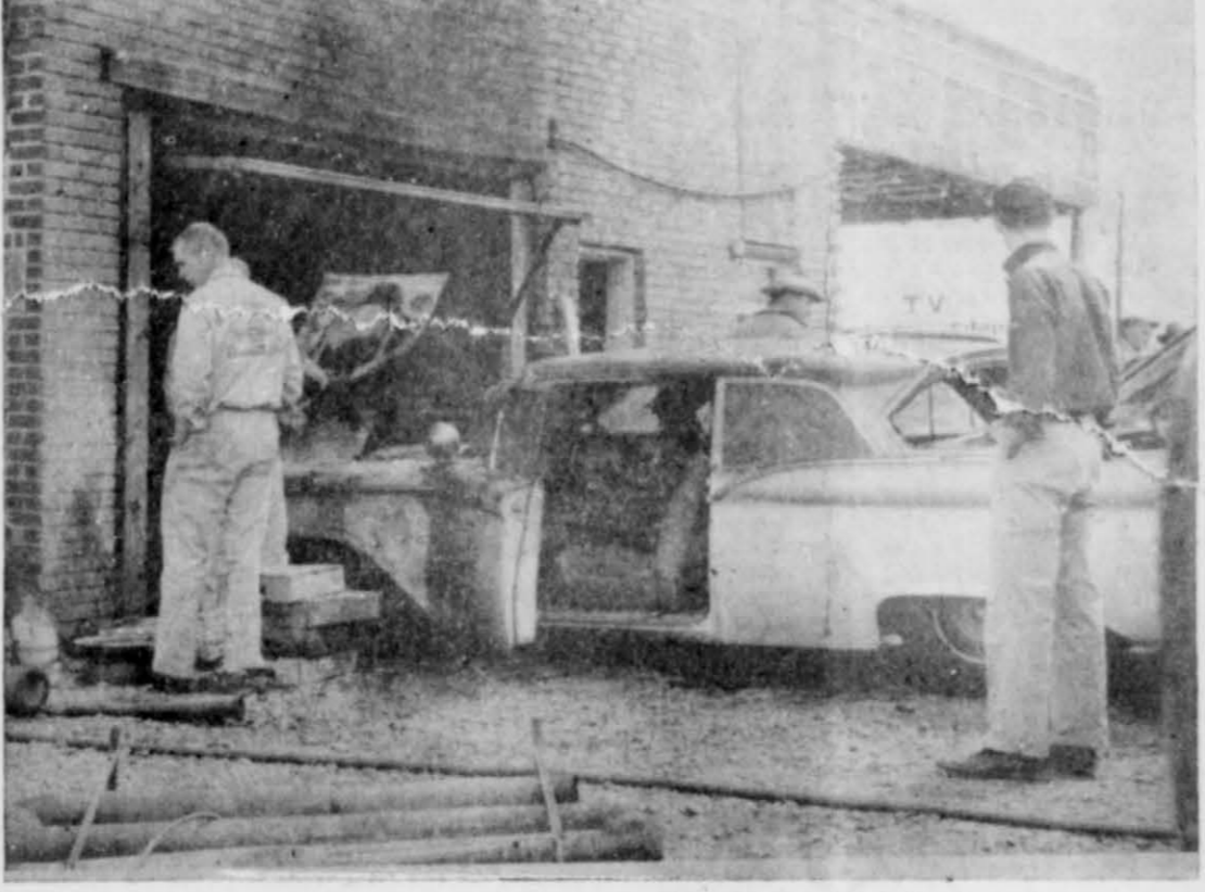
THIS HIGHWAY PATROL CAR was heavily damaged at 1 o'clock Wednesday afternoon when it caught fire while the motor was being cleaned with kerosene at the Magnolia Service Station at the corner of northwest Bedford and First Street. Cleaning the engine was Benze Espinoza, about 25, an employee of the station. The fire apparently was caused by a short under the hood since the motor was cool. One witness said the car's horn and siren started just before the fire boiled up. The station, owned by Choc Lay, also received considerable damage, with all the woodwork, including the roof, being burnt out of the washroom. Dollar estimates of the loss were unobtainable. —staff photo
