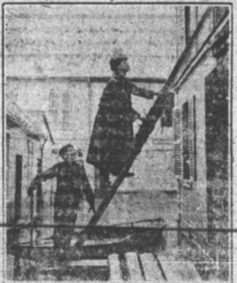
LADDERS USED TO REACH UPPER STORIES.
