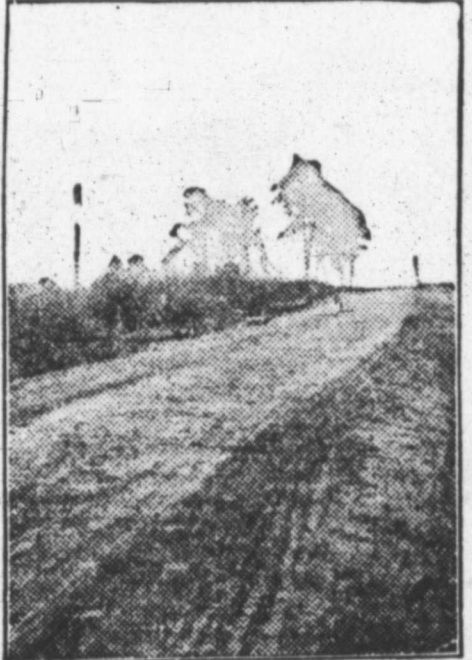
Virginia Road After Improvement With Top Soil Gravel.
