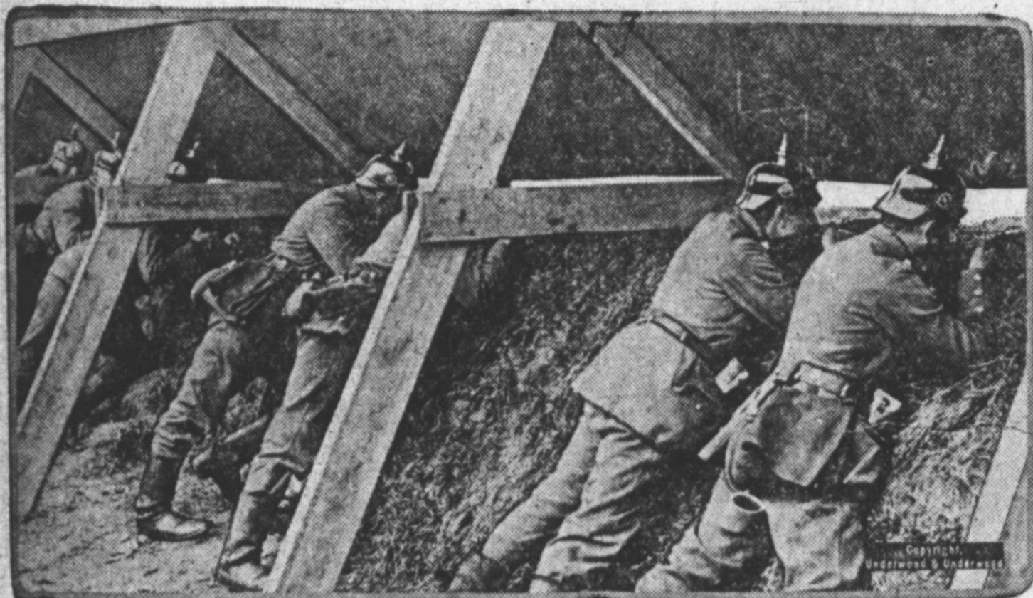
German sharpshooters behind such splinterproof sloping sheds as this are almost impossible to dislodge. From behind straw breastworks they fire through a narrow slit that runs the entire length of the shelter.
