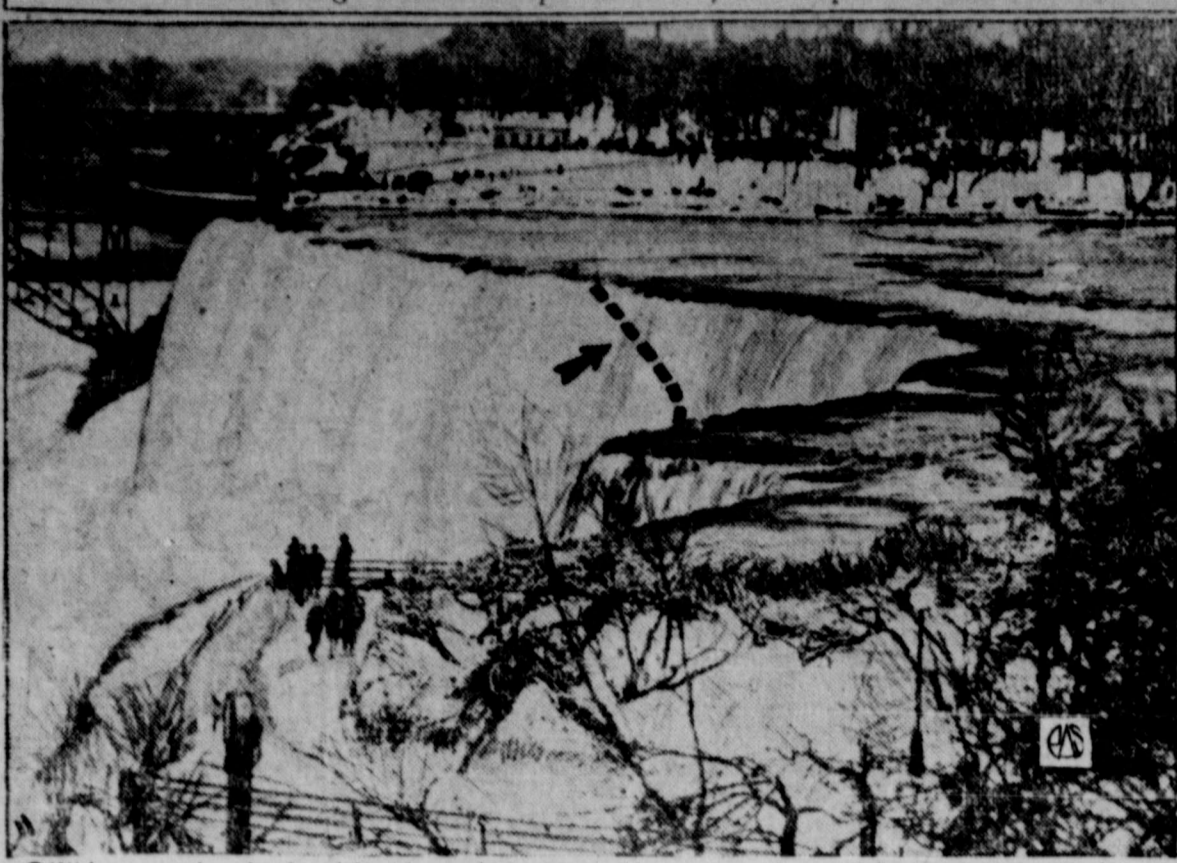
Without warning, in the night when nobody was looking, a huge chunk of limestone about 175 feet and 150 feet wide broke off the edge of the American Falls at Niagara and plunged into the gorge below the Falls. This changes the contour of the Falls completely, but without impairing their beauty. The rock is gradually wearing away but this is the largest single break in recorded history. The photograph was taken from Goat Island, looking toward the American side.
