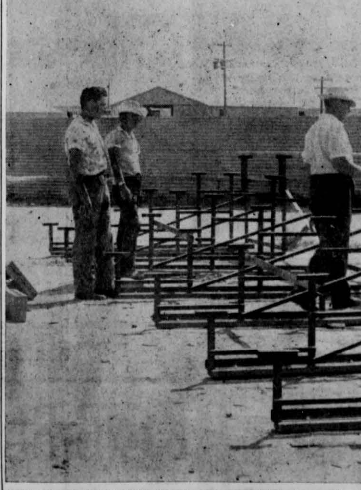
NEW BLEACHERS WERE INSTALLED TUESDAY at the Dimmitt ball park by Dimmitt JayCees. The new steel and wood bleachers were used to replace the old wooden ones due to the large crowds at the park since the Little League activity started. Cost of the low bleachers was about $400. —staff photo
