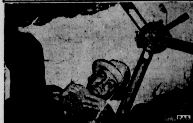
Here's a worm's-eye view of an avalanche in the making. Lowering himself into a huge fissure at the top of the "moving mountain" in Los Angeles' Elysian Park, a daring cameraman shows how the ever-widening crack is being checked hourly to determine course and extent of the next in a series of huge earth-slides that have already sent millions of tons of rocks, earth and trees tumbling 350 feet into Riverside Drive, Dayton Avenue, below, and even into the dry bed of the Los Angeles river, 1,000 feet away.
