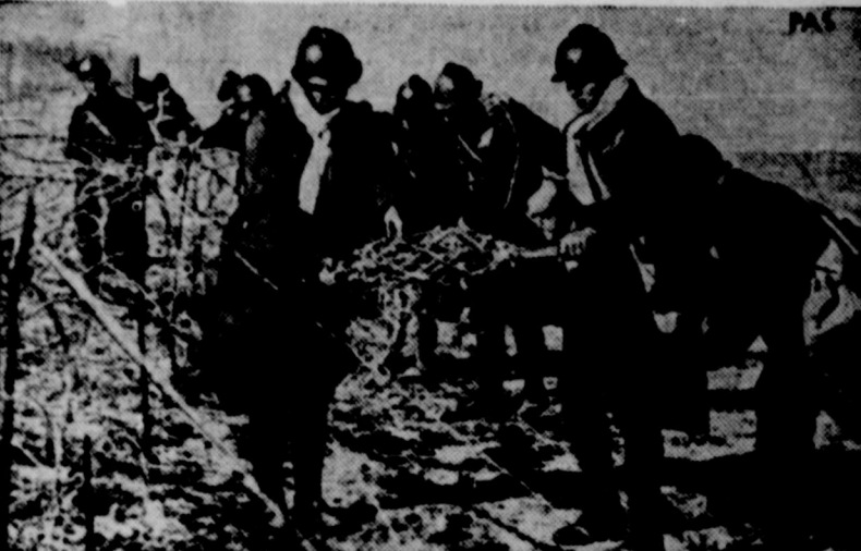
TUNIS, Tunisia . . . A detachment of soldiers string barbed wire before one of the new fortifications in the Mareth Line. The wire is strung on spikes which have been imbedded in blocks of concrete and buried in the ground.
