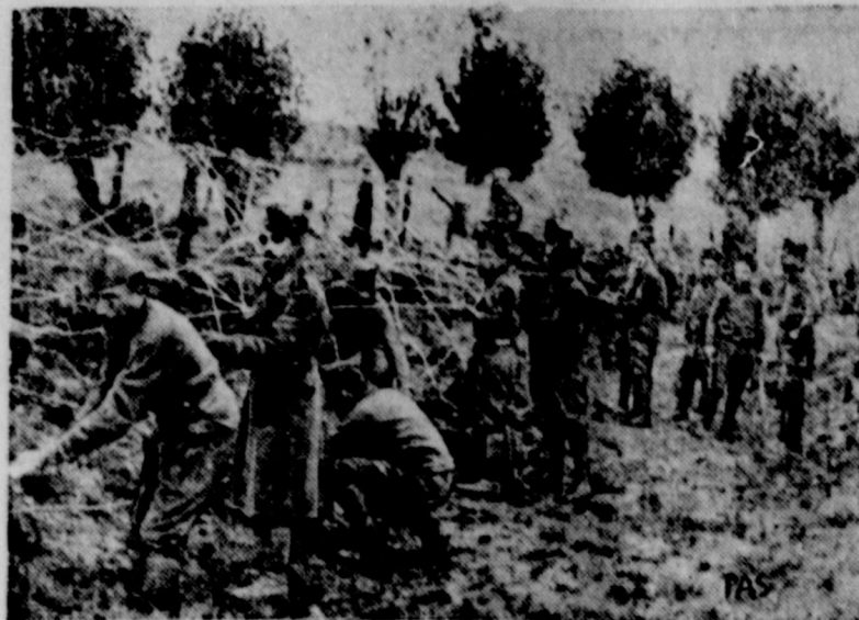
FRENCH FRONT . . . French soldiers erecting a defense network of barbed wire at the front. Photo passed by French censor.
