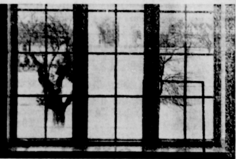
Here is one way to control that annoying fogging and condensation on the windows in your new home. Shown here are three casement windows. Notice that two of them are entirely clear because of inside double glazing. The other window has had the inside double glazing removed, with the result that it is fogged up almost immediately. When this picture was taken the inside room temperature was 71 degrees, while outside the thermometer stood at 15 degrees above zero.
