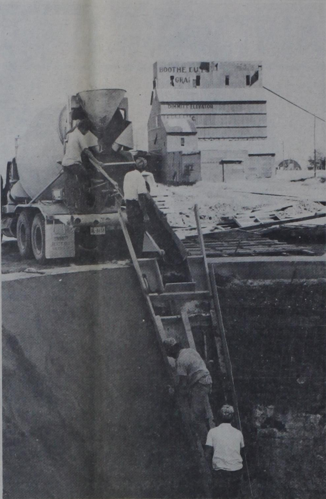
THE CHANGING SCENE is evident this week in Dimmitt's elevator district as a new elevator starts going up while the city's oldest remaining elevator comes down. In foreground, Dimmitt Ready Mix workers form the pit for a new elevator at WC Grain Co., between East Bedford and Jones Streets. In background, the old Boothe Elevator—built by C. W. Boothe in 1929—is being torn down. The Boothe Elevator was the second one ever built in Dimmitt; the first one burned down about 10 years ago.
