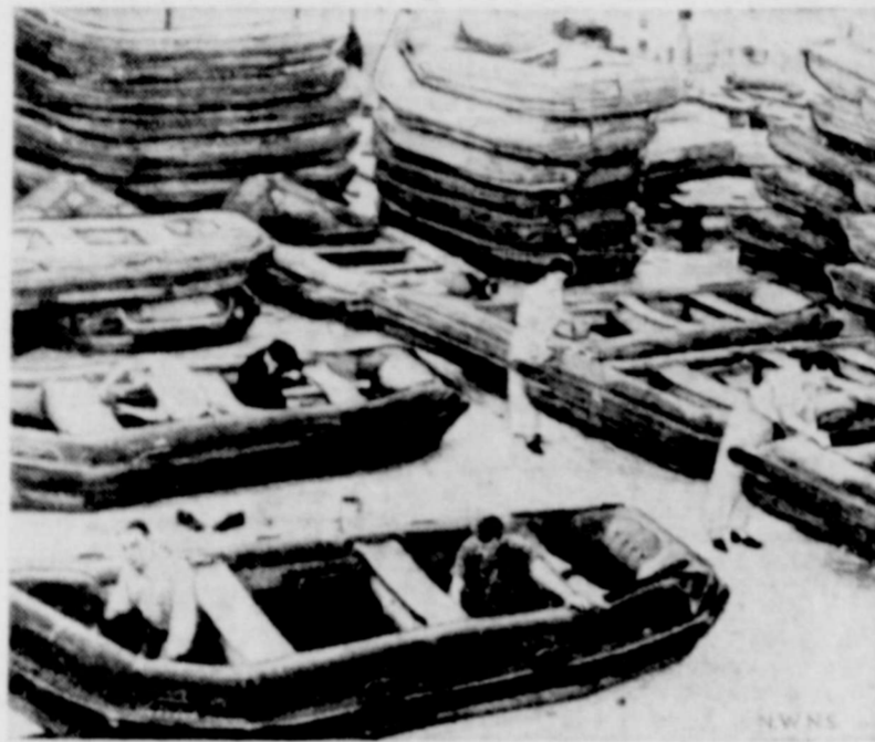
Rubber assault boats for the U. S. marines are shown in near-complete form at an Akron, Ohio, factory. Designed for tough, rugged, abusive service, these boats when deflated are the ultimate in compactness, and extremely light in relation to the loads they will carry. The U. S. war and navy departments, which approved this picture, are equipping both army and navy planes with them. Recently three U. S. navy fliers survived the crash of wind and waves through 34 days on one of these rubber rats.
