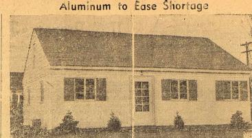
Houses like that pictured above, built of prefabricated aluminum panels, are being erected in Akron, Ohio, by the Goodyear Aircraft Co. Exterior surface is sheet aluminum attached to wood. Between the outer shell and inner fiberboard finish is layer of aluminum foil, serving as insulation. Sides and roof are coated with plastic paint, impregnated with asbestos. Upper section of house shown above is of wood, to demonstrate variety possible with this type of building.
