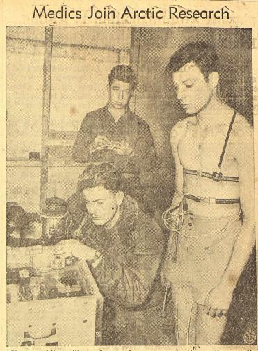
How a soldier will stand up under extreme Arctic weather condi-tions is being investigated, with the latest scientific devices, by Army medics with Task Force Williwaw at Adak, Aleutian Islands. Above, Capt. R. B. McGee, Altoona, Pa., operates a potentiometer attached to thermocouple harness worn by Pfc. Thomas Morgan, Roanoke, Va. Device registers temperatures in various parts of the soldier's body.
