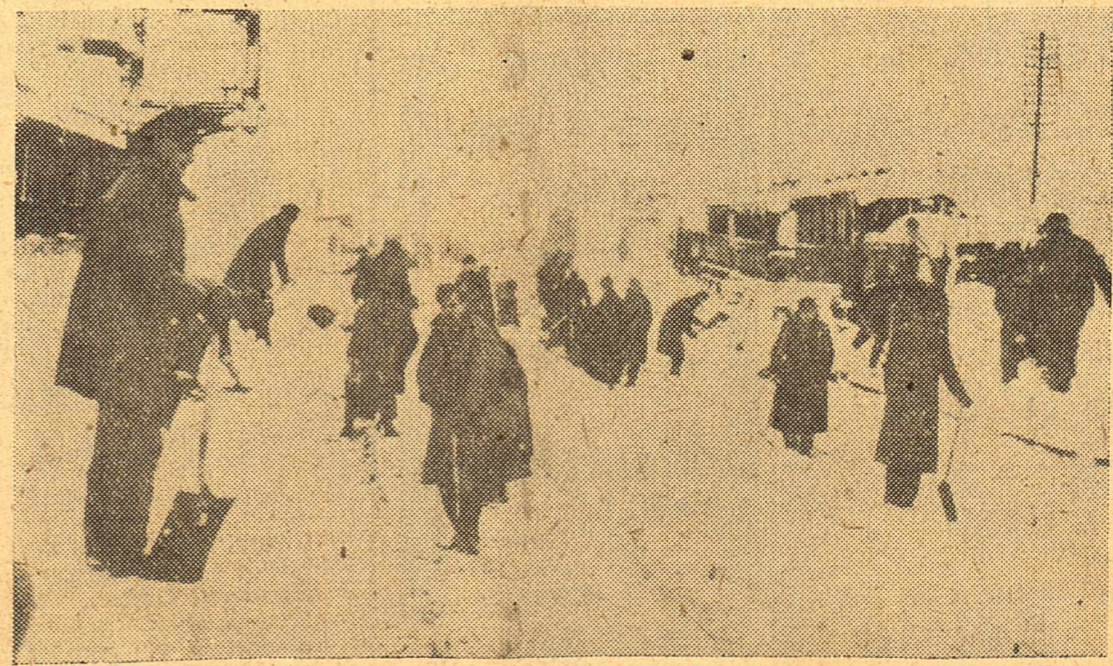
German prisoners of war working in bitter cold at Dunford Bridge, Yorkshire, England, clear the railroad tracks of snow after blizzards isolated this and other villages in the worst winter England has had for years.
