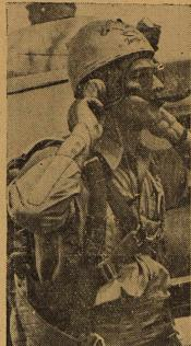
and crash helmet. Helmet contains ear phones and a tiny lip microphone so test pilot can talk with control tower.
