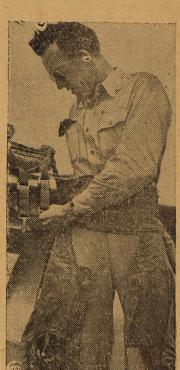
Test pilot Tony LeVier straps himself into a "G-suit" so he won't black out on sharp turns at near supersonic speeds. Bladders force blood driven downward by centrifugal force back into pilot's brain.
