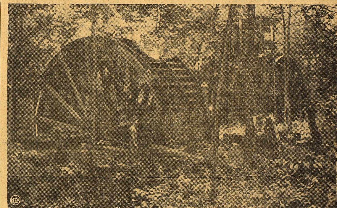
In Colonial days, these giant waterwheels powered the Ringwood Mines smelting furnaces. One of the wheels is more than 200 years old; it played a part in making cannon for "Old Ironsides."
