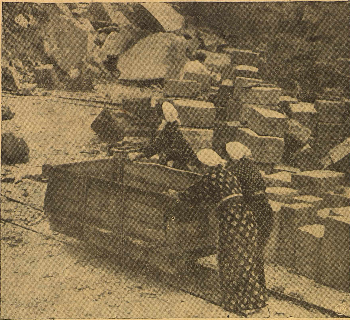
Clad in colorful kimonos, and barefooted, these Japanese women push a car along the rails in a rock quarry on Niijima Island, near Tokyo. Besides moving heavy loads of the huge granite blocks, the women mine them, using crude hand tools.
