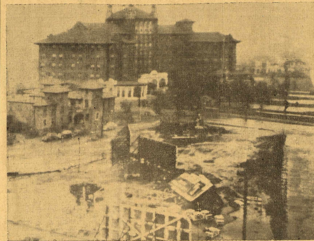
Wreckage of a watermelon parlor which was demolished when a 69-mile wind struck Galveston is shown in the foreground. The famed Galvez Hotel, in the background, was undamaged.
