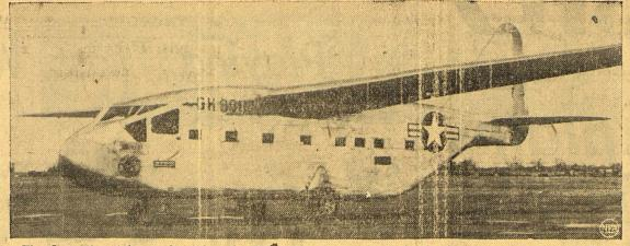
The first all-metal assault glider, the XC-18A "Avitruc," begins taxi and ground tests at Fort Dix, N. J., prior to its initial test hop over Trenton, N. J. America's largest glider, the craft was designed for use as a troop carrier for the airborne army of the future.
