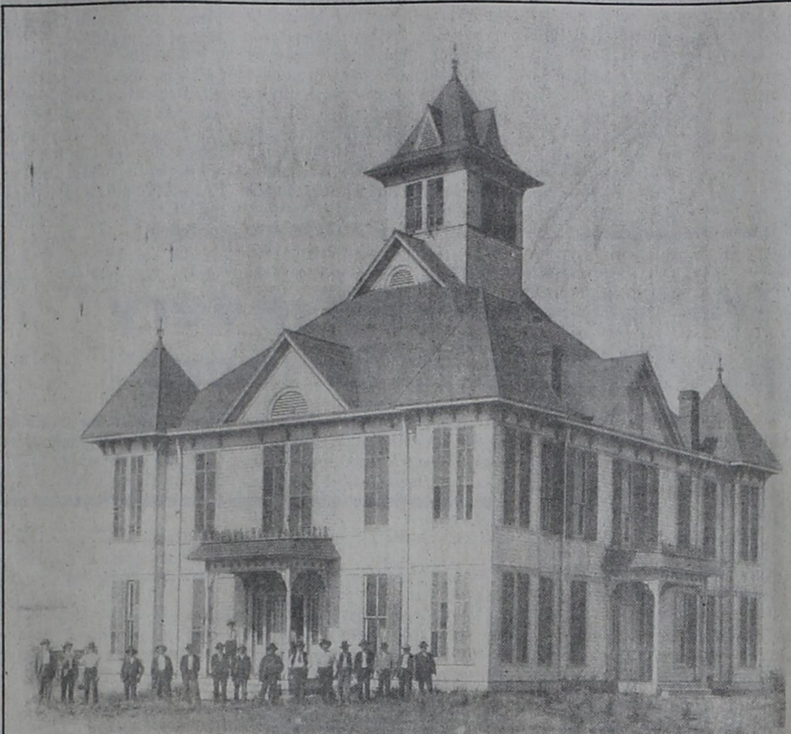
CASTRO COUNTY'S FIRST COURTHOUSE was completed in December, 1892, and served the county until it burned the night of August 26, 1906. The building was elaborate, with many decorations and other adornments. The cupola could be reached by ladder, and many poker games were held in the cupola. The
