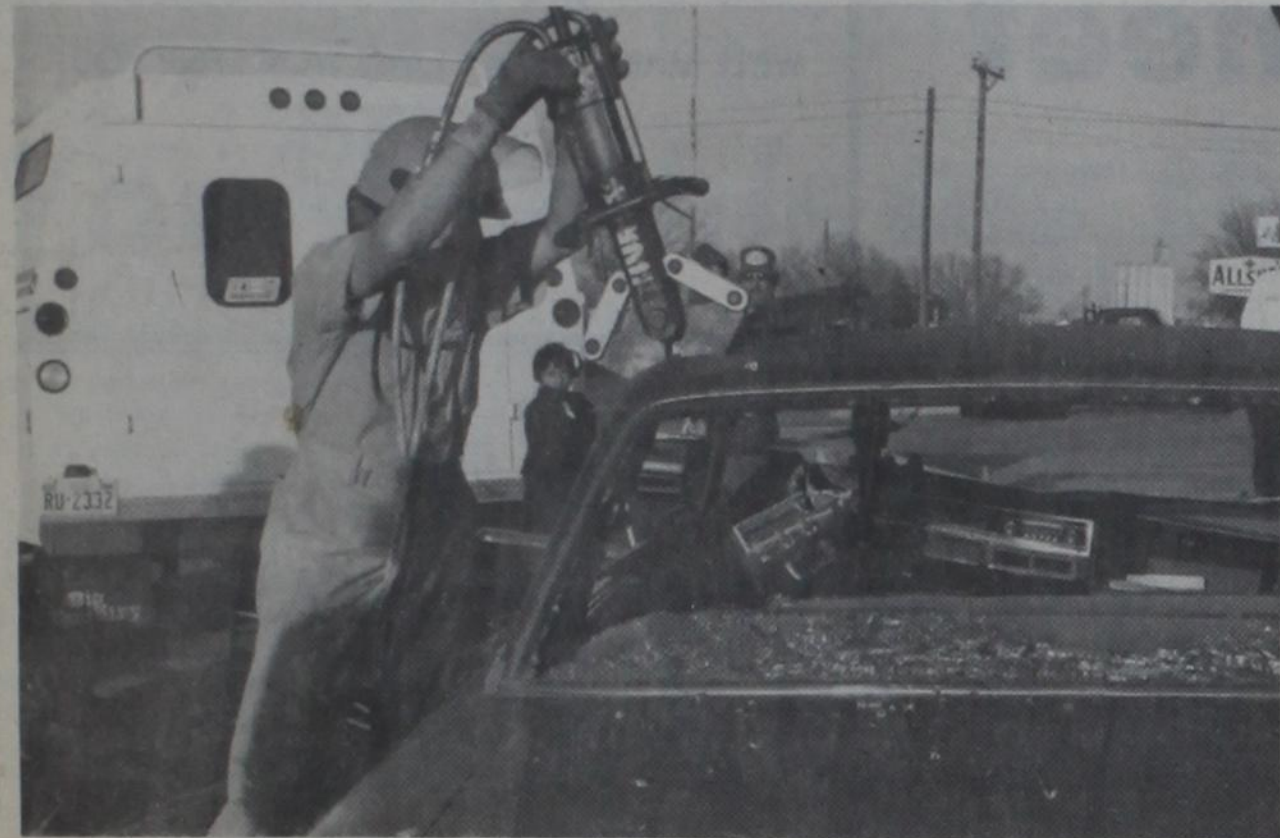
SWITCHING TO THE SHEARS , another component of the Hurst Rescue System, Gill cuts through the cab-frame of the car after having sheared the door-post. After a pair of similar cuts on the other side, Gill and one other man were able to fold the roof back, exposing the entire passenger compartment of the car. For good measure, Gill also used shears to snip off the steering column.
