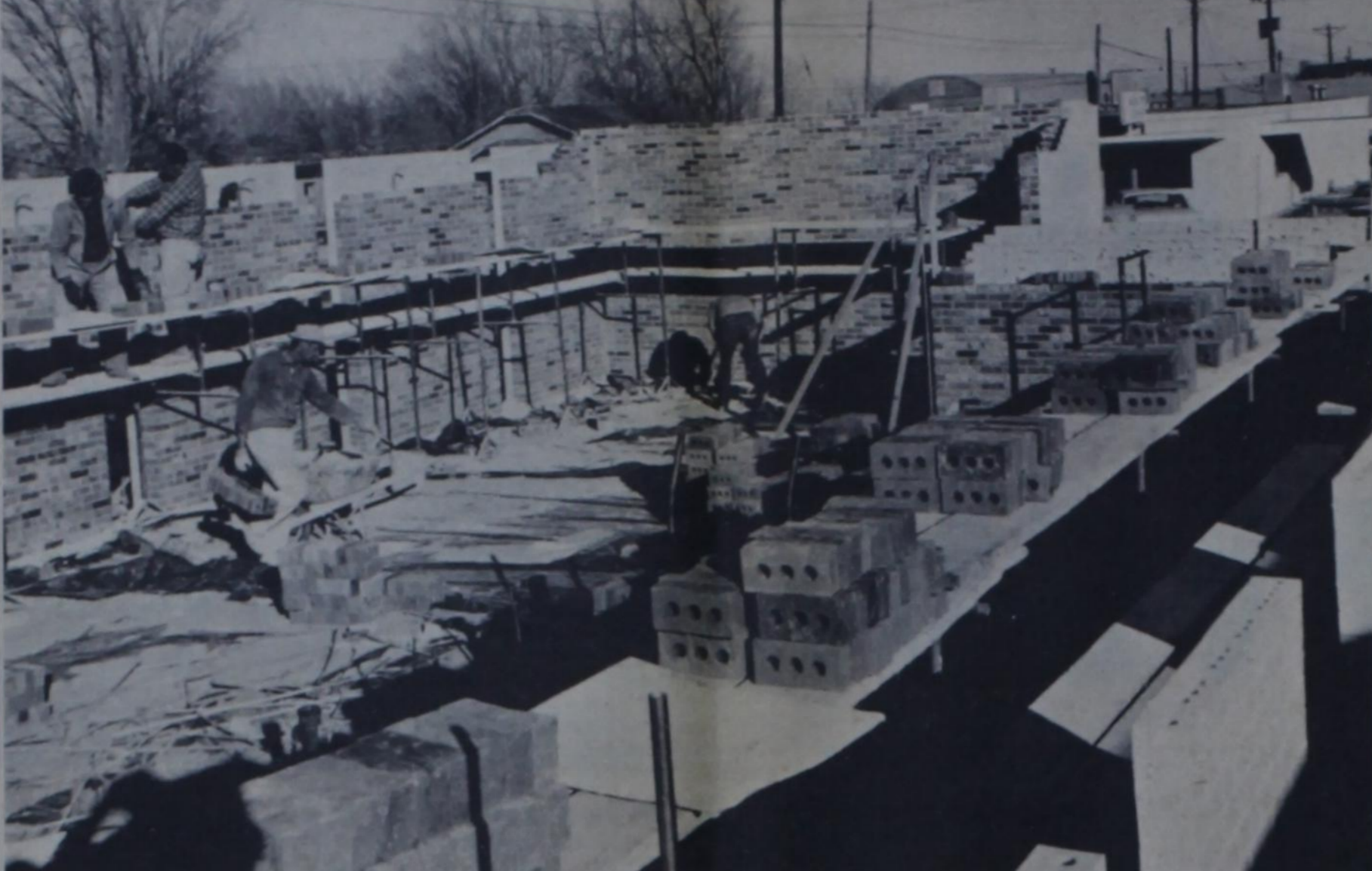
THE SCHAEFFER BUILDING at 103 NW Third St. is expected to be completed by latter February. The modern, 2,100 sq. ft. brick building is being built by Stanley Schaeffer for lease to Schaeffer & Harden, Certified Public Accountants. It features double brick wall construction with an exterior of glazed white brick and brick inner walls. The interior will feature paneled walls, draperies, carpet and terrazo flooring. Construction is by Dimmitt Ready Mix.
